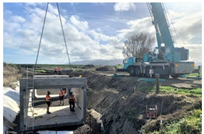
Culvert crossing construction WAIKATO REGIONAL COUNCIL
