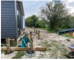
Tansy Bliss helping concrete the deck piles KEITH WOODLEY
