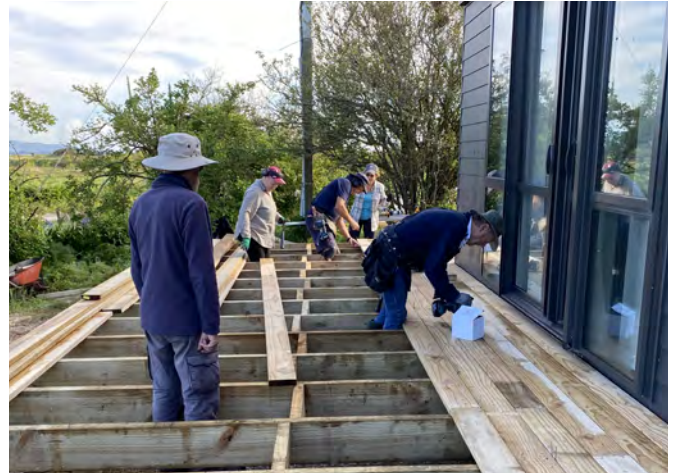
Deck building volunteers KEITH WOODLEY
