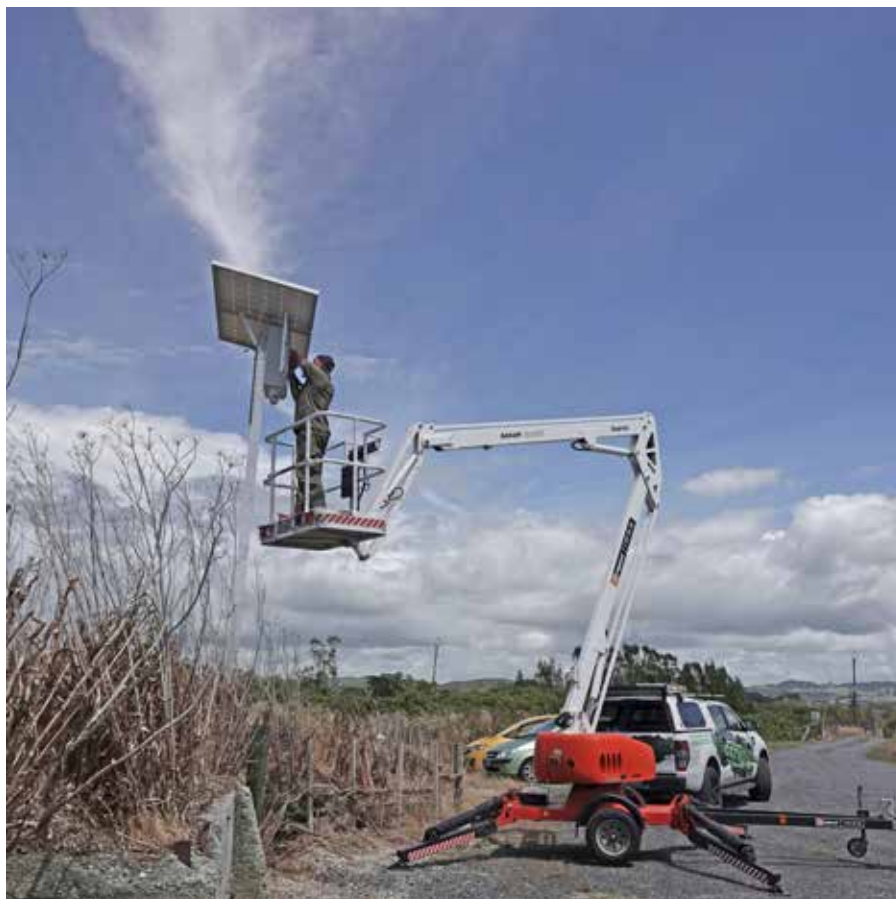
THIEVES BEWARE: A security camera has now been installed above the carpark at the Findlay Reserve. There have been fewer thefts from cars so far this summer and it is hoped that the camera, along with existing steps such as asking visitors to close the gate behind them, will remove the problem altogether. Photo / Jim Eagles
