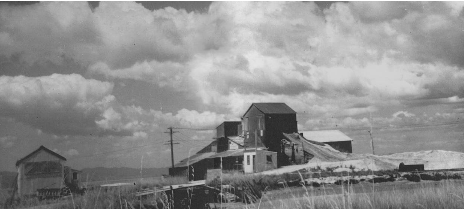
The Limeworks as it was in the late 1950s. Photo Noelle MacDonald
